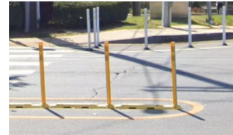
Pavement Markings & Flex Posts
